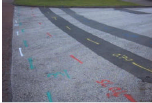
Fig. 4 Marking on the site of existing utility networks
