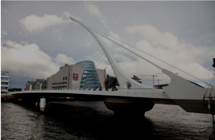
Figure 8. Samuel Beckett bridge, Dublin
