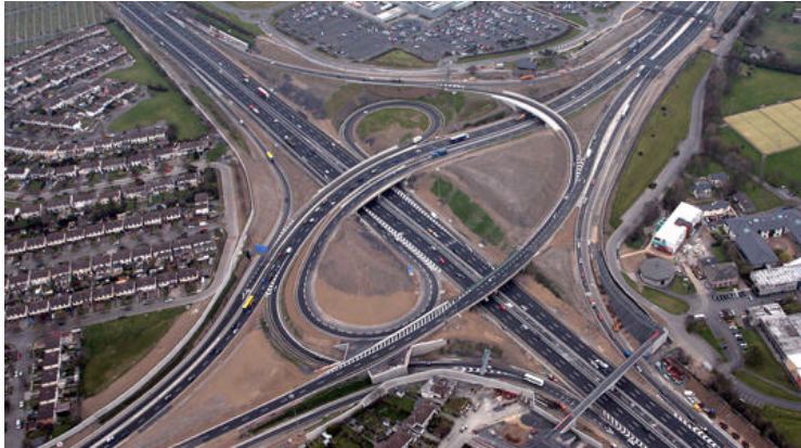
Figure 3. Road junction on the M3 motorway Dublin
