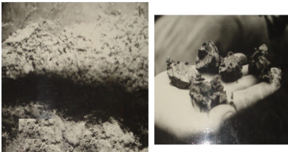
Figure 4. Frontal view of the soil part with lateral failure and clay fragments from the dislocated area.
