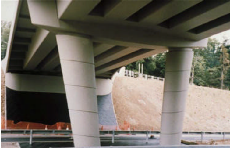
Figure 3. Killarney road bridge piers
